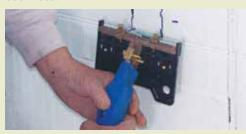
**STEP 1:** Select the position for your box. Using a hot-knife or cutting tool, cut the opening in the EPS foam.
