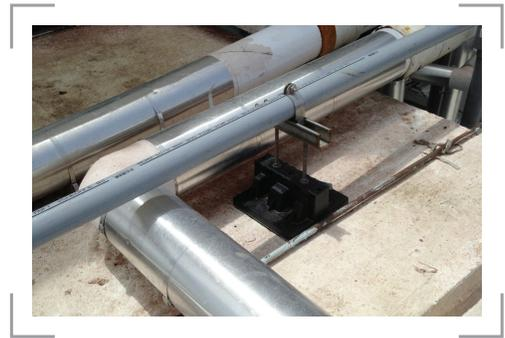
Roof Top Blox are designed specifically as roof supports to be used on commercial roof piping support and platform support applications.
