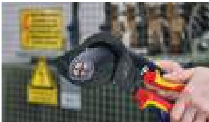
Cross-section of a steel wire armored cable
