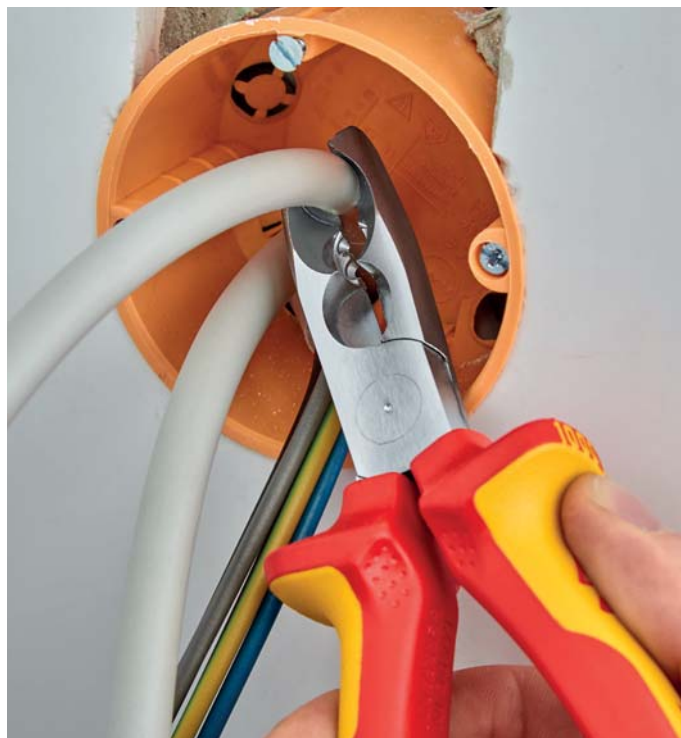
Stripping cable inside deeply mounted flush sockets
