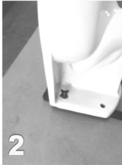
2 Install supplied wing nuts.
