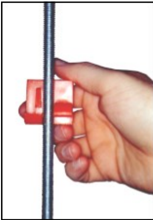
Place hanger around rod as shown.
