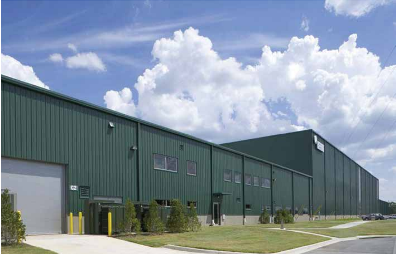
REHAU production plant, Cullman, Alabama
