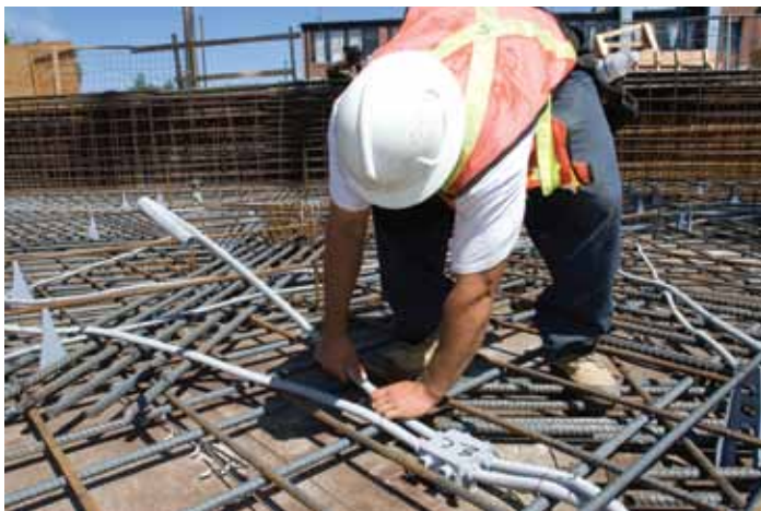
Diagram 3. ENT pipe and fittings in a High-Rise application.
