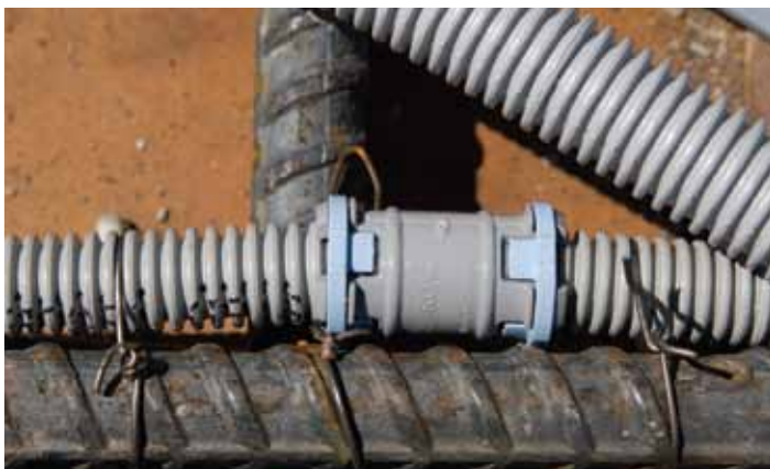
Diagram 1. ENT pipe attached with a coupling and tied to a rebar.
