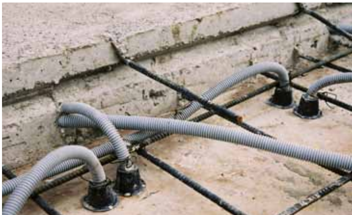
Diagram 2. ENT encased in a concrete application.
