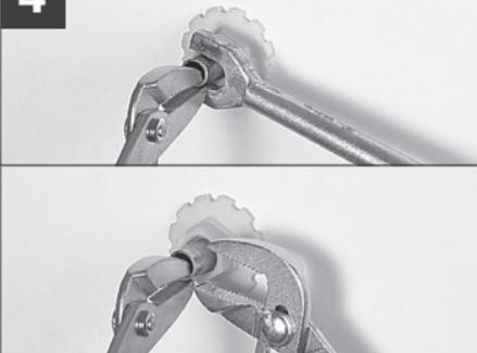
Insert nose of first pliers into copper tube and hold firmly. Swing a second pair of pliers or a shower arm tool, levering off first pair of pliers to push Shower WallNut firmly against finished wall.
