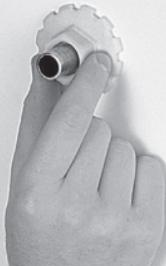
Cut excess copper stub out off leaving exactly  $1\frac{1}{2}$ " to finished wall. Deburr the cut end, then push Shower WallNut over the tube.
