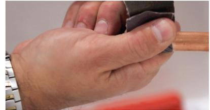
**3.** Thoroughly clean inside and outside of copper tube to remove all burrs.
