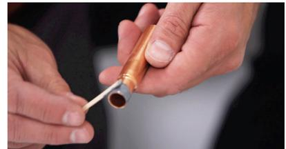
**6.** Working quickly, apply epoxy completely to outside of reduced end of copper extension.
