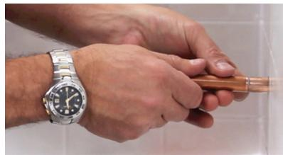
**8.** Insert copper extension into tube in wall and wipe away excess epoxy on exterior of tube.
