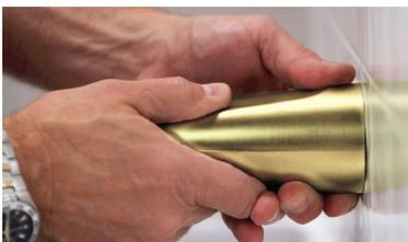
**1.** Remove old spout; clean the copper tube to remove burrs; clean the wall surface around the spout.
