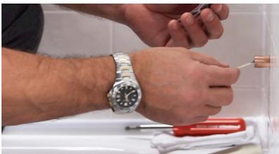
**7.** Apply epoxy completely to inside of tube in wall.
