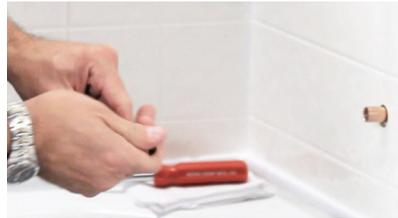
**2.** Remove any old fittings with hacksaw, making sure to leave at least a 1¼" length of copper tube exiting the wall.
