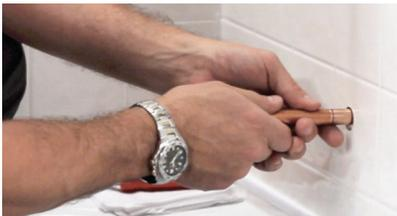
**4.** Dry fit copper extension to make sure it fully slips into copper tube in wall.
