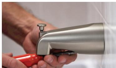
**5.** Tighten the screw to secure the SmartSpout snug to the wall. Do NOT over tighten as the wall could become damaged.
