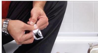
**5.** Squeeze one side of epoxy pouch to burst the middle seal. Work epoxy to other side and mix thoroughly until gray color appears.
