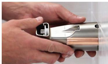
**2.** Mark the copper stub out even with the hash mark on the underside of the SmartSpout and cut off excess pipe.
