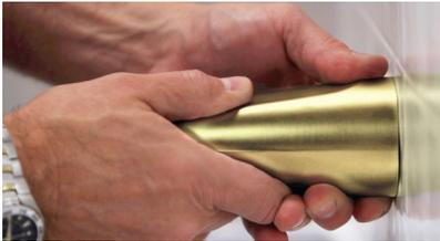
**1.** Remove old spout; clean the copper tube to remove burrs; clean the wall surface around the spout.
