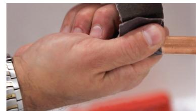
**3.** Thoroughly clean inside and outside of copper tube to remove all burrs.
