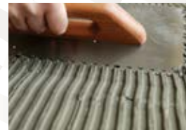
THINSET MORTAR APPLICATION
