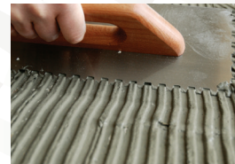
THINSET MORTAR APPLICATION
