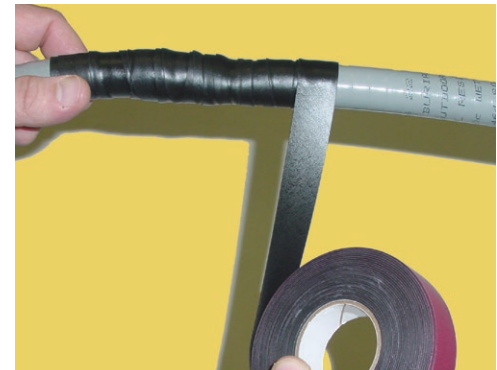
Tape will create a sealed protective covering
