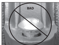
OVAL NECK OF BOLT NOT SEATED PROPERLY
