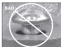
OVAL NECK OF BOLT NOT SEATED PROPERLY
