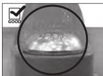
OVAL NECK OF BOLT SEATED PROPERLY
