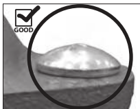
OVAL NECK OF BOLT SEATED PROPERLY
