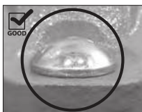
OVAL NECK OF BOLT SEATED PROPERLY
