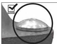
OVAL NECK OF BOLT SEATED PROPERLY
