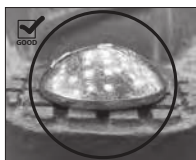
OVAL NECK OF BOLT SEATED PROPERLY
