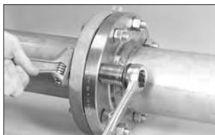
4-Bolt Tightening Pattern
