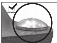
OVAL NECK OF BOLT SEATED PROPERLY
