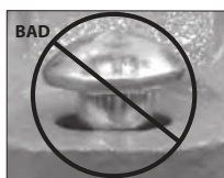
OVAL NECK OF BOLT NOT SEATED PROPERLY
