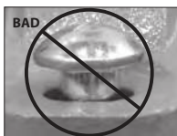
OVAL NECK OF BOLT NOT SEATED PROPERLY
