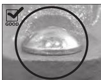
OVAL NECK OF BOLT SEATED PROPERLY
