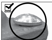
OVAL NECK OF BOLT SEATED PROPERLY
