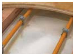
Our LockDown fastener is designed specifically for under-floor PEX applications. Its loose hold allows PEX to move during expansion and contraction of the tubing. The LockDown won't pop open like other similar clips you may have seen or tried. Use LockDowns for attaching 3/8" or 1/2" PEX; do not use it for 5/8" PEX as it will fit too tightly. Order five LockDowns for 10' of PEX. Follow all Installation Guidelines carefully.
