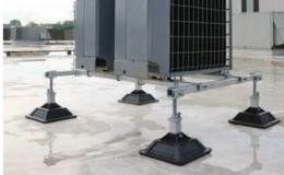
Pyramid rooftop supports are a surface mounted solution for supporting electrical and mechanical applications on a variety of roof surfaces.
