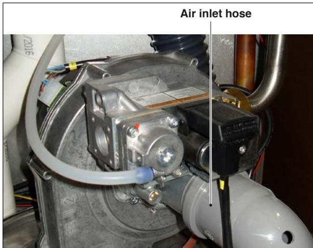
Fig. 64 Air inlet hose SSB160
