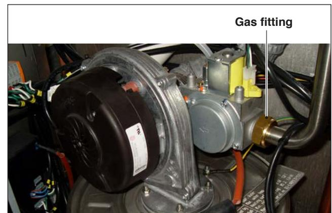
Fig. 48 Gas fitting - model SSB85 - SSB120
