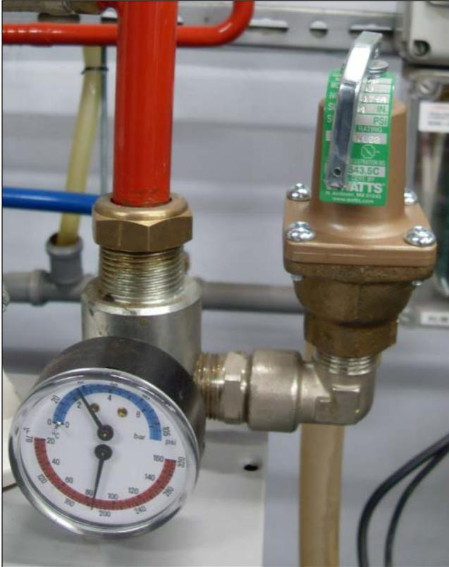
Fig. 22 Pressure relief valve (pipe connection from boiler supply to relief valve is field supplied and does not come with the boiler).
