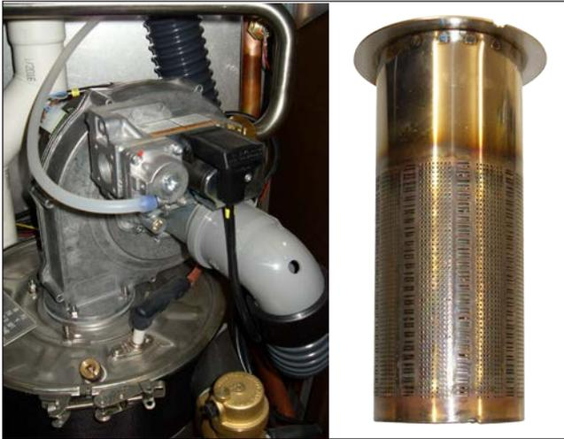
Fig. 4 Burner head
