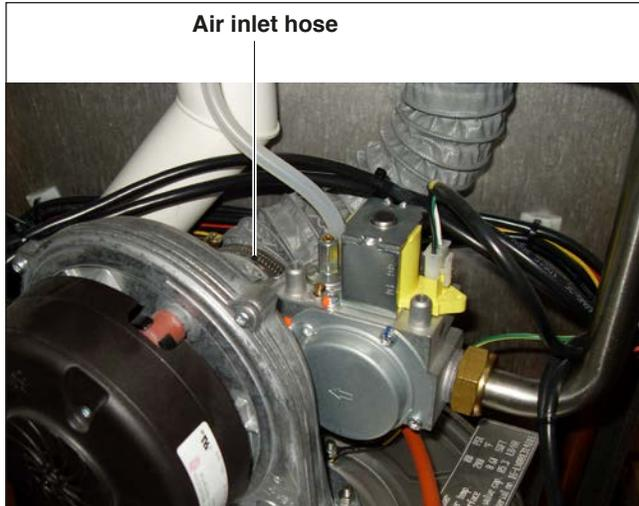
Fig. 63 Air inlet hose SSB85 - SSB120
