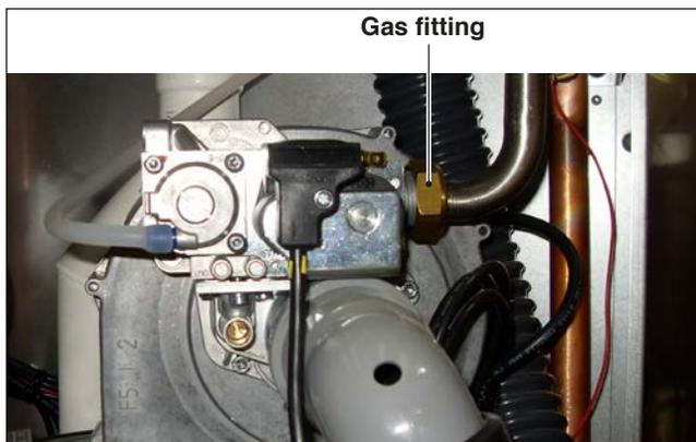
Fig. 52 Gas fitting - model SSB160
