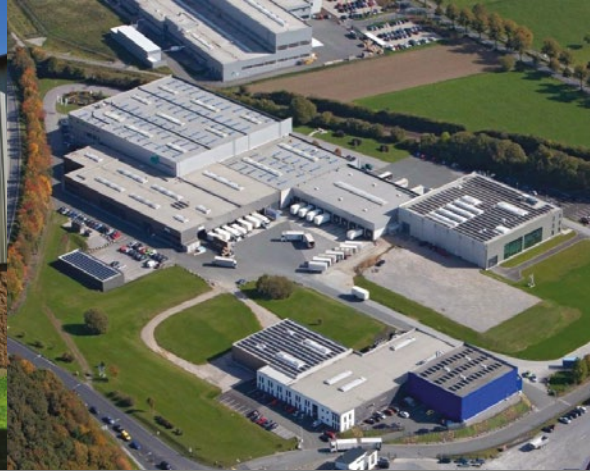
Centrotherm Systemtechnik GmbH Brilon, Germany
