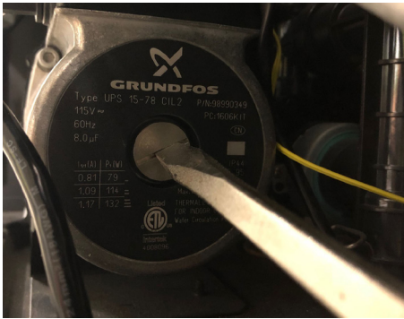
Figure 54 - Bleeding the Internal Pump
