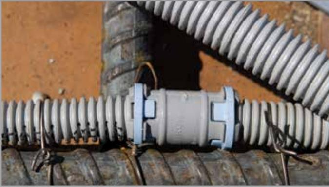
Diagram 1. ENT Pipe Attached with a Coupling and Tied to a Rebar
