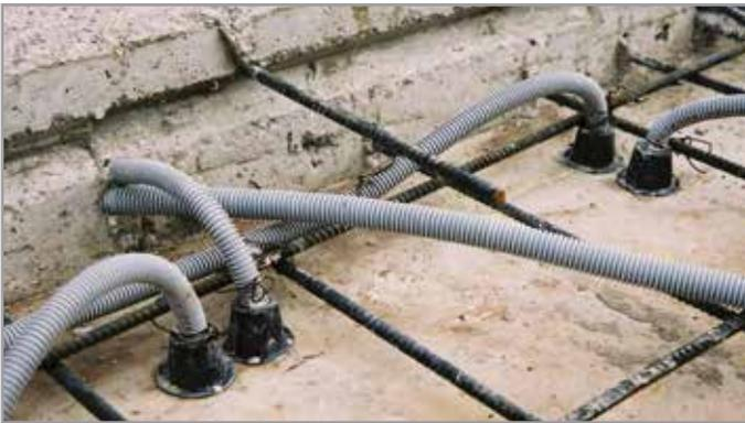
Diagram 2. ENT Encased in a Concrete Application
