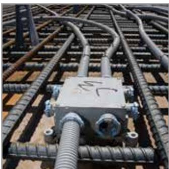
**NAPCO Slab Boxes Hubs are Elevated to Permit a Larger Diameter Rebar**
