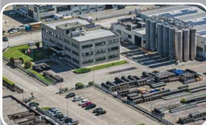
Production Facility - Castel Guelfo di Bologna (BO)
