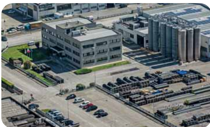
Production Facility - Castel Guelfo di Bologna (BO)
