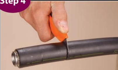
Carefully, finish cutting through the sleeve down to the stainless corrugated pipe using a sharp utility knife.
