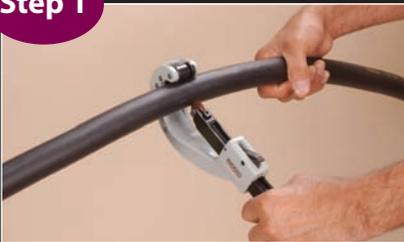
Unroll pipe into trench or on the ground and cut to desired length – plus one foot. Cutting up to 1" can be done with a large tubing cutter. For 1 1/4" – 2" sizes, a reciprocating saw is recommended.
