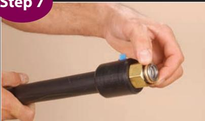
Remove adapter and split rings from fitting. Attach adapter to equipment. Slip coupling and nut over end of pipe all the way to expose first corrugations of pipe. Insert split rings into first corrugation as shown.
