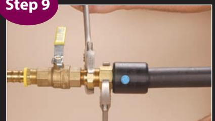
Thread the nut onto adapter previously installed on the equipment. Using appropriate wrenches, hold adapter and tighten nut to proper torque specified. Do not overtighten or use any thread sealants on this connection. This is a metal-to-metal seat and will not seal if pipe dope or thread sealants are used. Sealants are to be used on the NPT connection to the equipment only!
