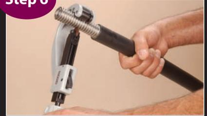
Using the tubing cutter, trim corrugated pipe to strip length specified on the Strip Length Chart shown above. Cut slowly in the root of the corrugation in the same manner you would cut copper tubing. Inspect end of pipe for a clean cut without tears in corrugation.
