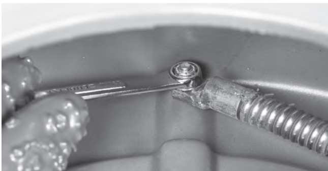
Figure 30 – Pigtail Anchor Bolt
