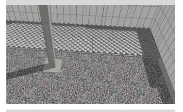
Step 7 Continue to place the rows of panels maintaining a staggered running bond layout.
