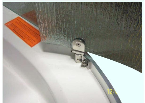
STEP 19: Tighten the Top Hinge (5) the same way as in the step 18.
