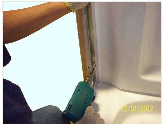
STEP 5: Place a level against the Wall Jamb and make sure the Wall Jamb is plumb. Mark the middle and top hole drill locations.
