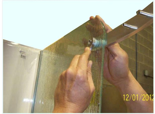
STEP 16: Mount Hinges (5) on the Door Panel (8), top and bottom. Reference Detail View II - Hinge Assembly(5) on page 4 of Exploded View.
