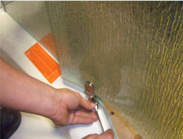
STEP 33: Apply clear mildew resistant silicone on the outside of tub shower from the top to bottom of the Wall Jamb (1, 1A).
