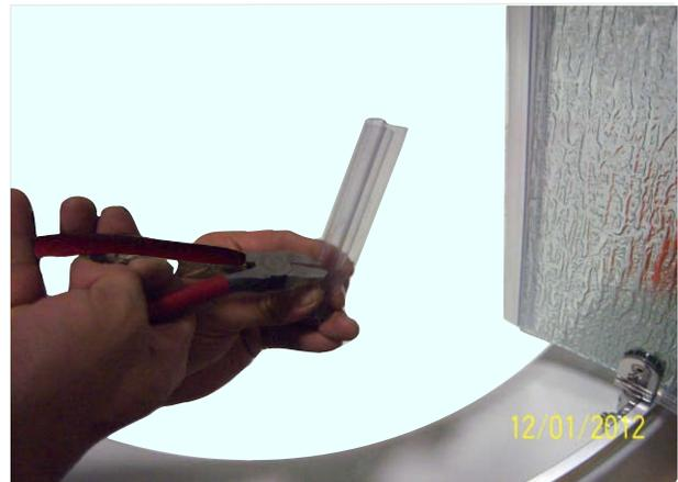
STEP 25: Insert Short Bottom Sweep Gasket Seal (15) onto the Door Panel (8) bottom glass as shown.
