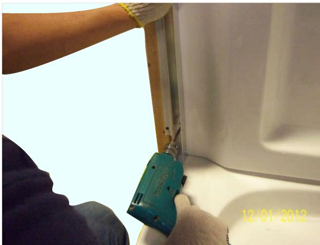
STEP 4: Using a Long Screw # 8 x 1" (11) provided, fasten the Wall Jamb (1) to the wall.
