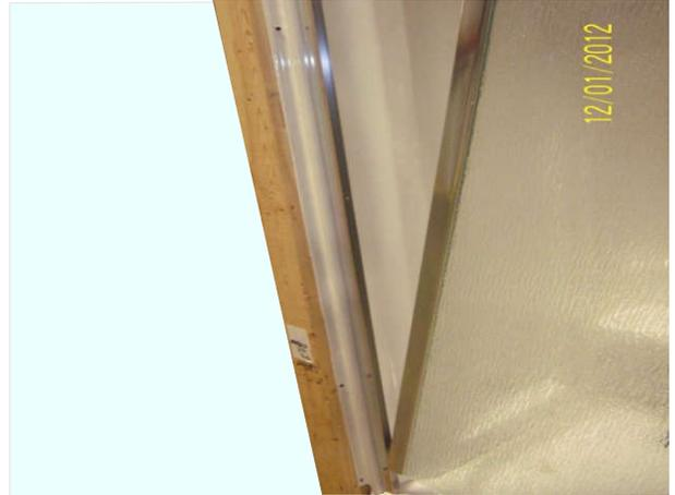
STEP 10: Insert Right Hand Fixed Panel (2A) into the Wall Jamb Right (1A). Repeat steps 8 - 9 on the right side.
