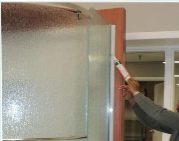
STEP 35: Finished Door Installation. If the door leaks make sure that it was sealed with clear mildew resistant silicone as specified in the installation manual.
