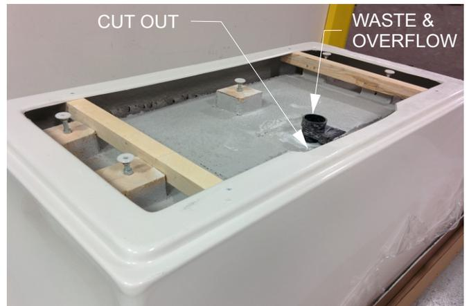
STEP 7: Lift the tub back into the correct position, levelling the tub if necessary (tub levelled at factory). Level by loosening the hex nut and threading the rod into or out of the block. Tighten the hex nut against the wood block once the foot is level. Connect the plumbing once the tub is level.
