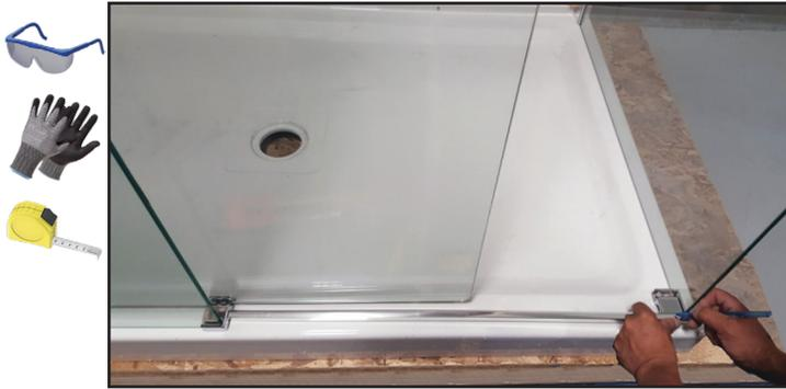
14. Slide up Corner Guide Block (RTC 7). Apply clear mildew resistant silicone underneath Sill (RT 6). Insert Sill (RT 6) in to the sill track of left Center Guide Block (RT 7).
