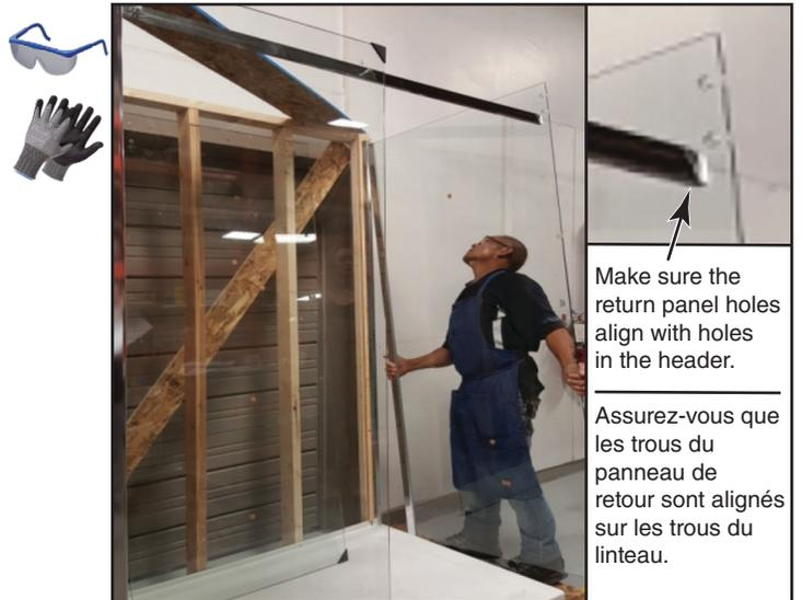
9. Install Header Bracket (RT 9) on the end of Header (RT 8) and attach the bracket to the Return Panel glass (RT 3).
