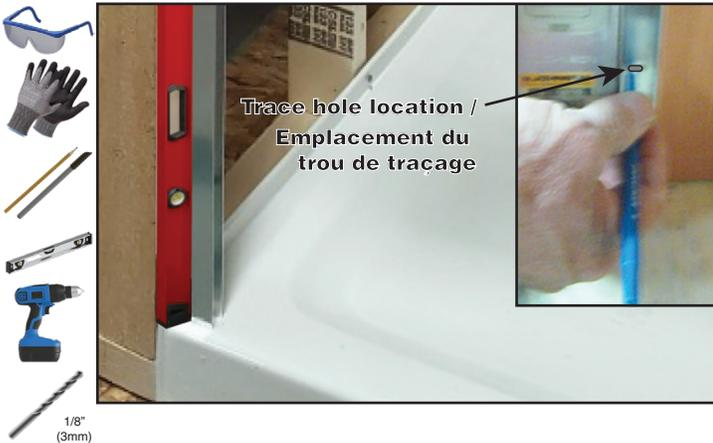
3. Screw Wall Jamb (RT 1) to the shower wall using  $1 \frac{1}{4}$ " (32mm) Screws (RT 14) at the bottom, middle and the top.
