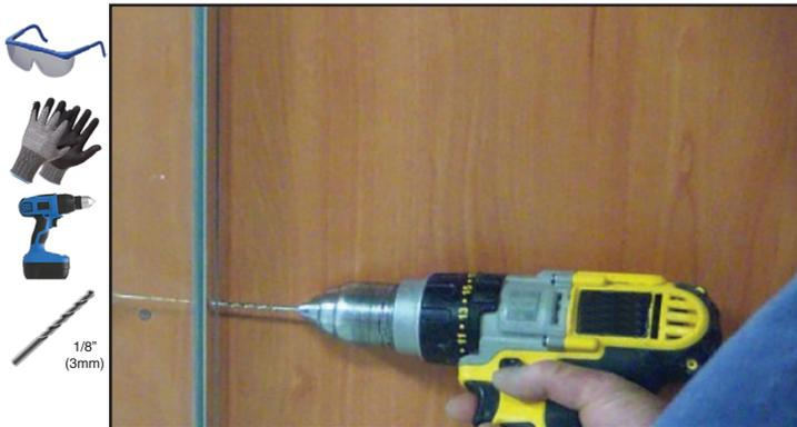
16. Screw Front Fixed Panel (RT 4) and Return Panel (RT 3) to the Wall Jamb (RT 1) using Screws - 5/8" (RT 15) and Plastic Washer (RT 19) at the bottom, middle and the top. Cover Screws with Chrome Cap 1/2" diameter (RT 17).
