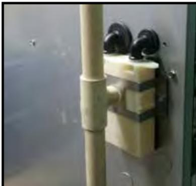
4. If extra security is desired, it is recommended to secure a strip of strapping around the drain. Utilize the existing condensate trap screws to secure the strapping.
